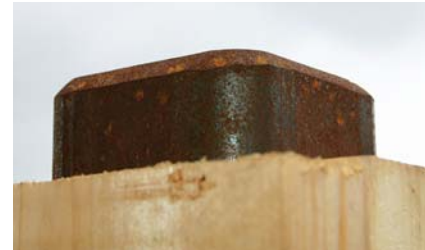
Figure 5. Wood cladding on the underside of the perimeter beam (left) precluded the use of bolting flanges for the columns. Instead, they're direct-welded. Beveled edges on the tops of the columns (below) expose the full thickness of the tubing wall for an optimal welded bead.
