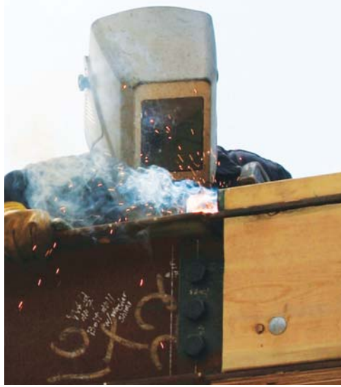
Figure 3. The drift-punch handle of a rigger's wrench aligns beams for bolting (left). Though bolting alone is sufficient, the author likes to add a couple of tacks to the joints to eliminate all possibility of movement (center). At welded perpendicular joints, the beams are coped for a snug fit (right).
