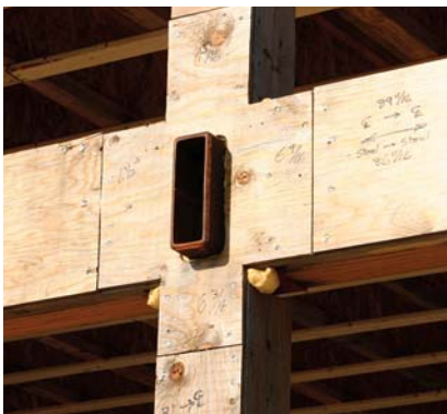
Figure 11. Three projecting steel beams support the wood I-joint framing in this 7-foot-deep roof overhang (top). A cantilevered shading trellis (center) projects from the western face of the house, attached to the steel posts by welded butt connections (above left and right).
