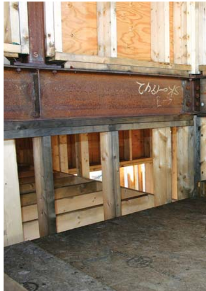
Figure 10. Web stiffeners at column locations are critical to preventing distortion of the beam flange during welding (left). Stainless steel shims help plumb second-floor columns (above).
