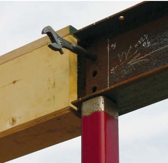
Figure 3. The drift-punch handle of a rigger's wrench aligns beams for bolting (left). Though bolting alone is sufficient, the author likes to add a couple of tacks to the joints to eliminate all possibility of movement (center). At welded perpendicular joints, the beams are coped for a snug fit (right).
