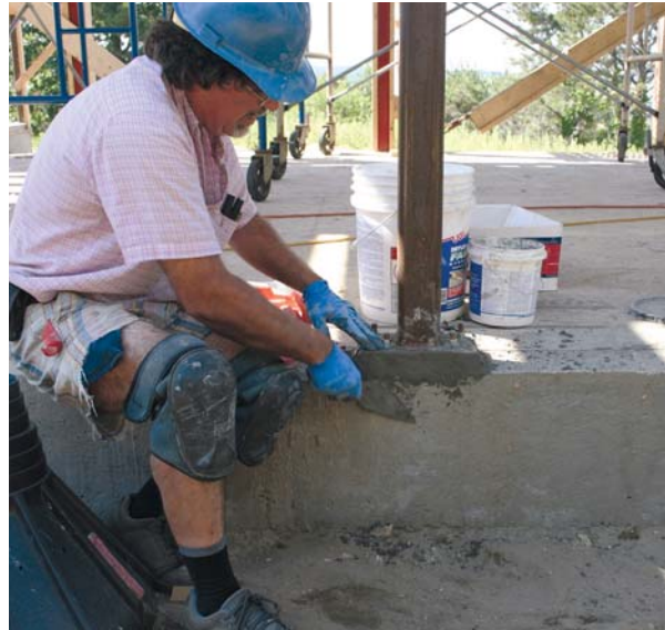
Figure 2. The moment frame begins at the foundation. MDO templates ensure that the holes in the column baseplates match the bolt holes in the concrete (above). The baseplates rest on setting nuts (above right), which are used to plumb the column and adjust it to finished elevation. The top nuts rigidly hold the columns in place. After the complete frame is assembled, the author packs the voids under the plates with fast-setting hydraulic cement (right).
