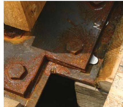
Figure 10. Web stiffeners at column locations are critical to preventing distortion of the beam flange during welding (left). Stainless steel shims help plumb second-floor columns (above).
