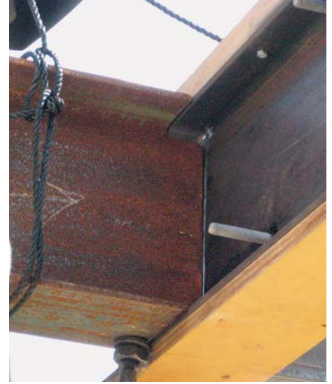
Figure 3. The drift-punch handle of a rigger's wrench aligns beams for bolting (left). Though bolting alone is sufficient, the author likes to add a couple of tacks to the joints to eliminate all possibility of movement (center). At welded perpendicular joints, the beams are coped for a snug fit (right).
