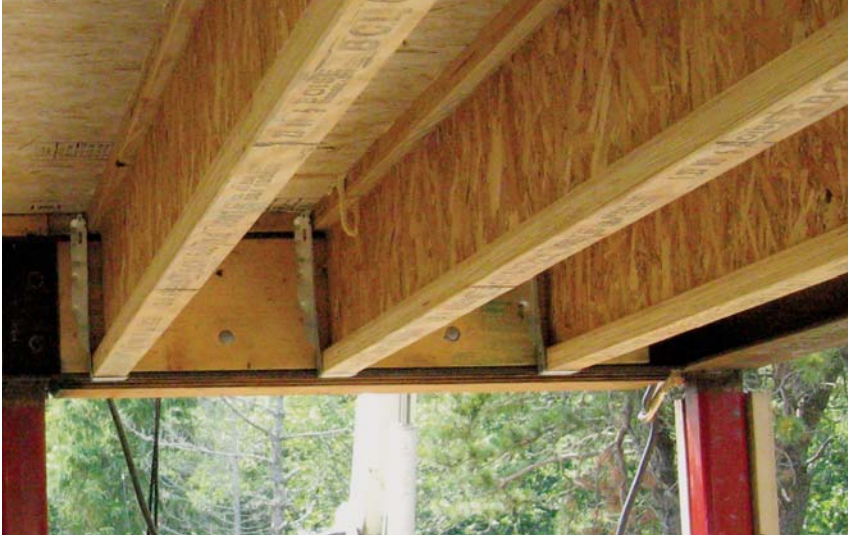
Figure 5. Wood cladding on the underside of the perimeter beam (left) precluded the use of bolting flanges for the columns. Instead, they're direct-welded. Beveled edges on the tops of the columns (below) expose the full thickness of the tubing wall for an optimal welded bead.
